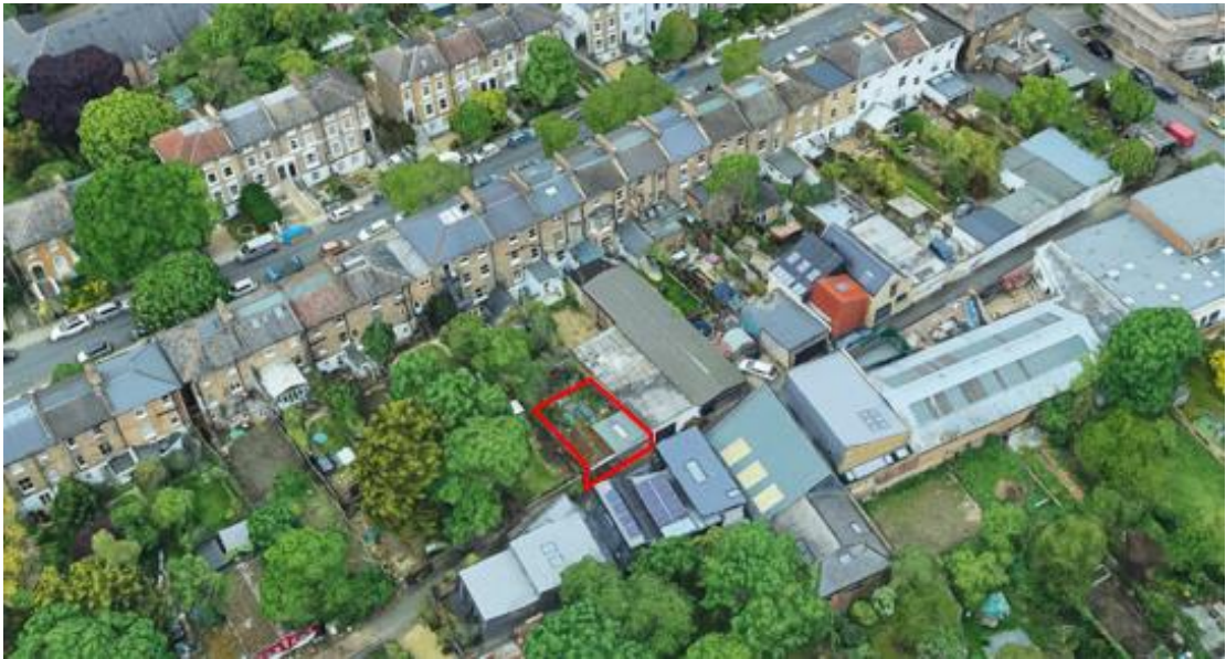
Photograph 1: Aerial photograph of site
