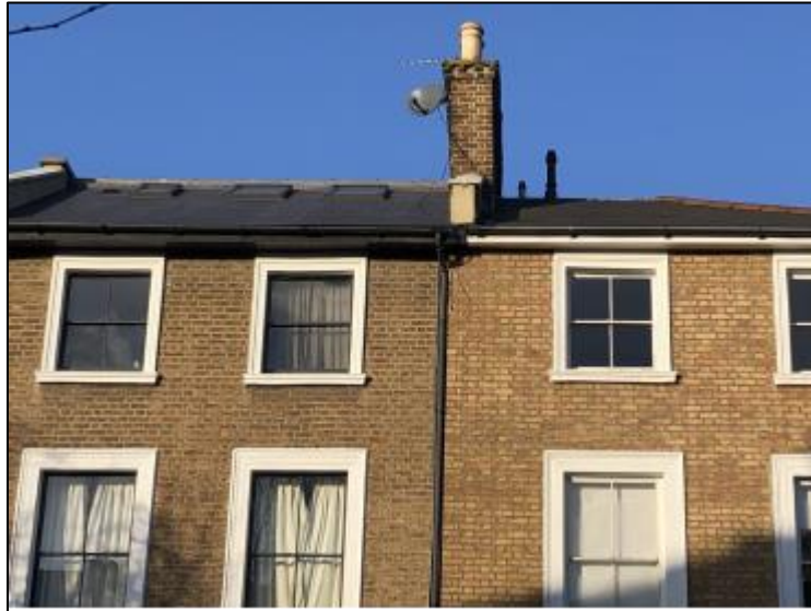
Photo 1. Front roof slope of No.16 Manor Avenue
