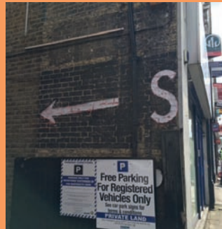
WWII SHELTER SIGNS e.g. Dartmouth Road, Forest Hill
