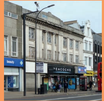
CIVIC, CULTURAL AND COMMERCIAL BUILDINGS e.g. 1920s commercial building on Lewisham High Street and in Catford Town Centre
