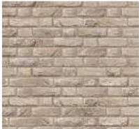
1 Buff brick in Flemish Bond
