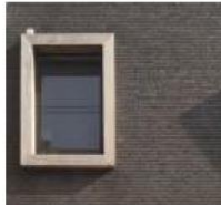
7 Timber window surround
