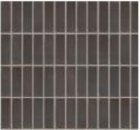
4 Dark brick in stack bond
