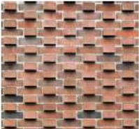
3 Recessed buff brick header detailing
