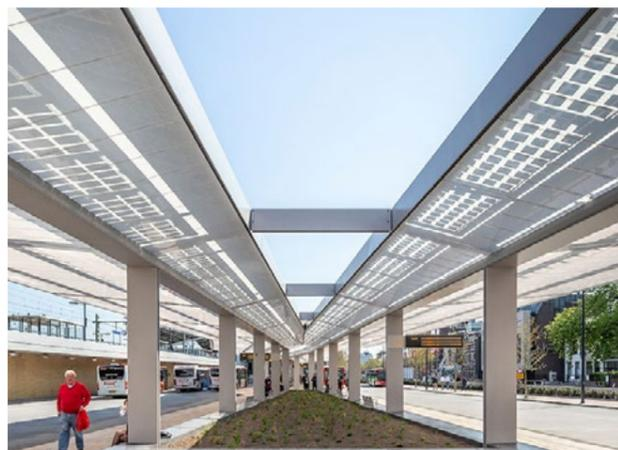
The newly designed Tilburg Bus Station by Cepezed in The Netherlands features a triangular, minimalistic circuit and uses an ETFE-foil for its awning cover. The positions of the bus are organized around its outer side where six are for boarding, and one is for de-boarding. 250m<sup>2</sup> solar panels supply Tilburg Bus Station with energy for the lighting, digital information signs, and heating of the waiting benches and staff room etc.
