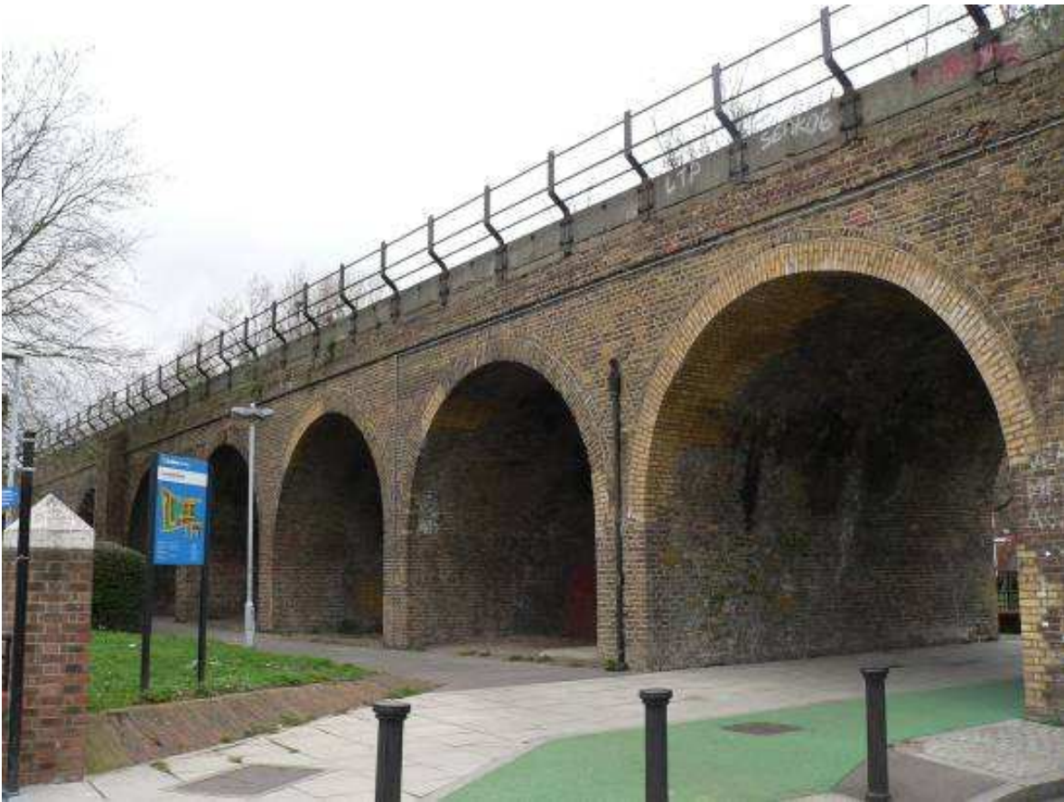
A section of the listed 1838 railway viaduct
