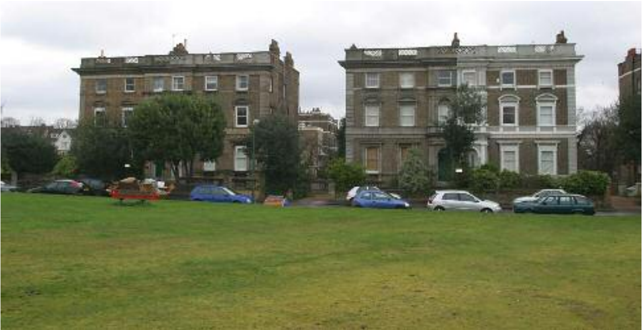
From left to right: No. 6 & 5 and 4 & 3 Aberdeen Terrace before works were carried out, date unknown (before May 2009, photograph submitted by the agent for a LBC application in 2009)
