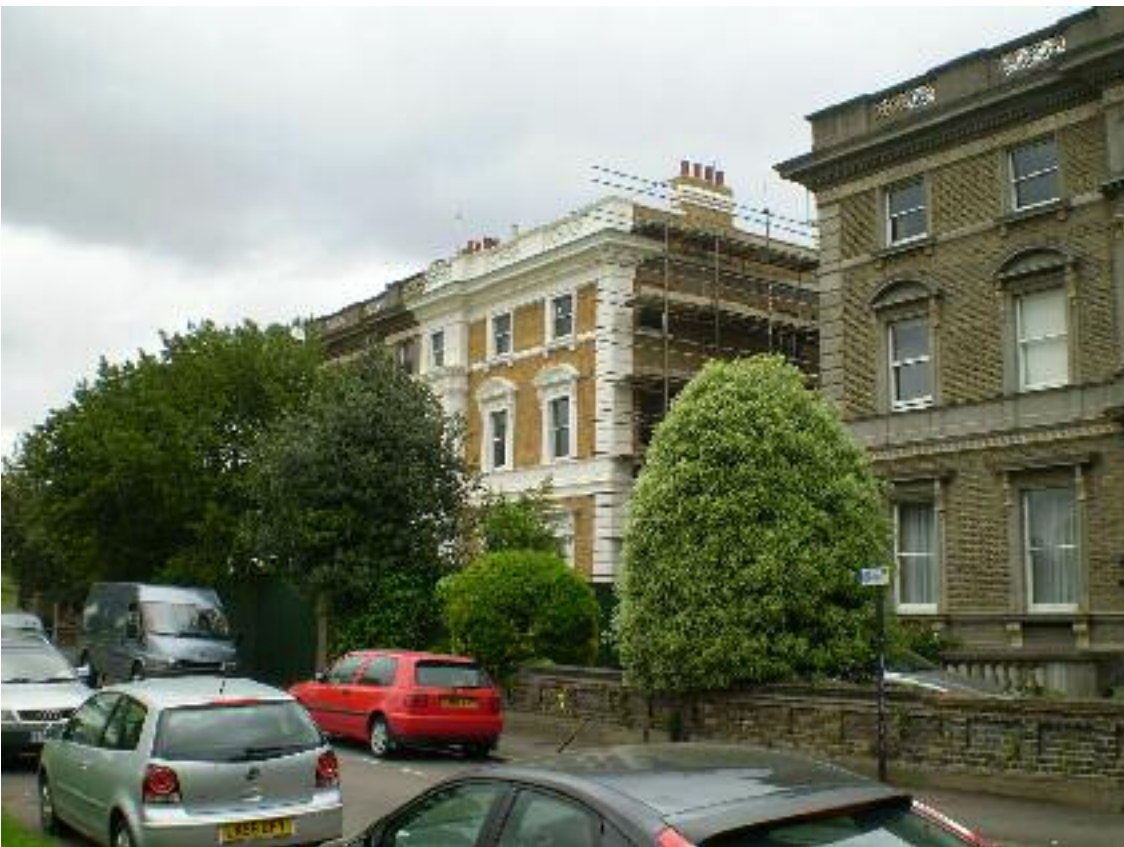
No. 5 Aberdeen Terrace after painting and cleaning, photograph taken 9.05.2009
