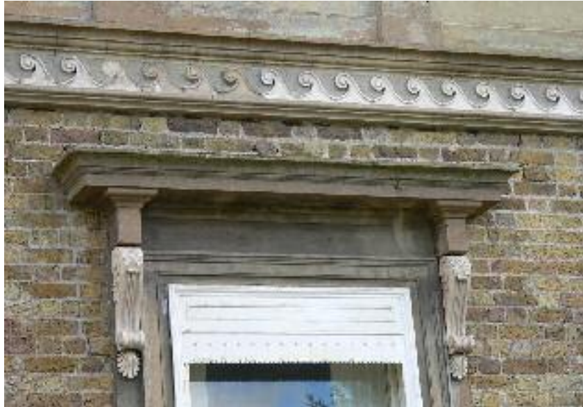
Stucco window surround with terracotta consol brackets and stucco frieze above with Vitruvian Scroll ornament at No. 6 Aberdeen Terrace (photograph taken 7.10.2010)
